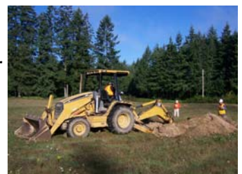
The design team digging test holes to sample soils.
